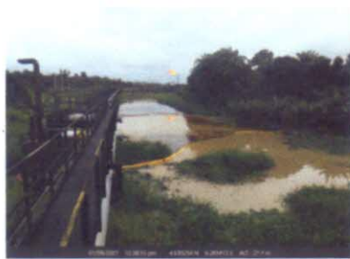
Fig B: Containment booms was deployed
